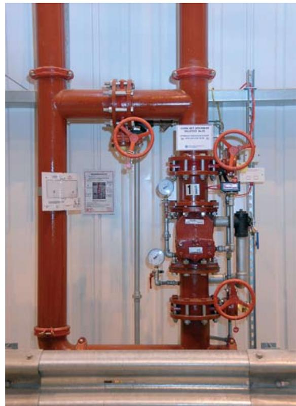
**Figures 61 and 62** Parts of a sprinkler system
