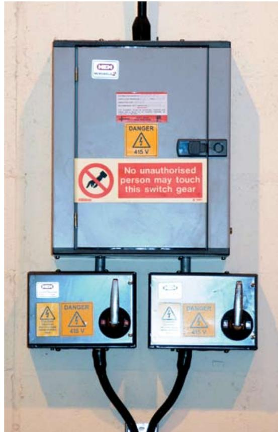
**Figure 10** Isolation switch for fixed equipment
