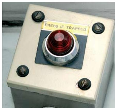
Figure 55 Trapped man alarm
