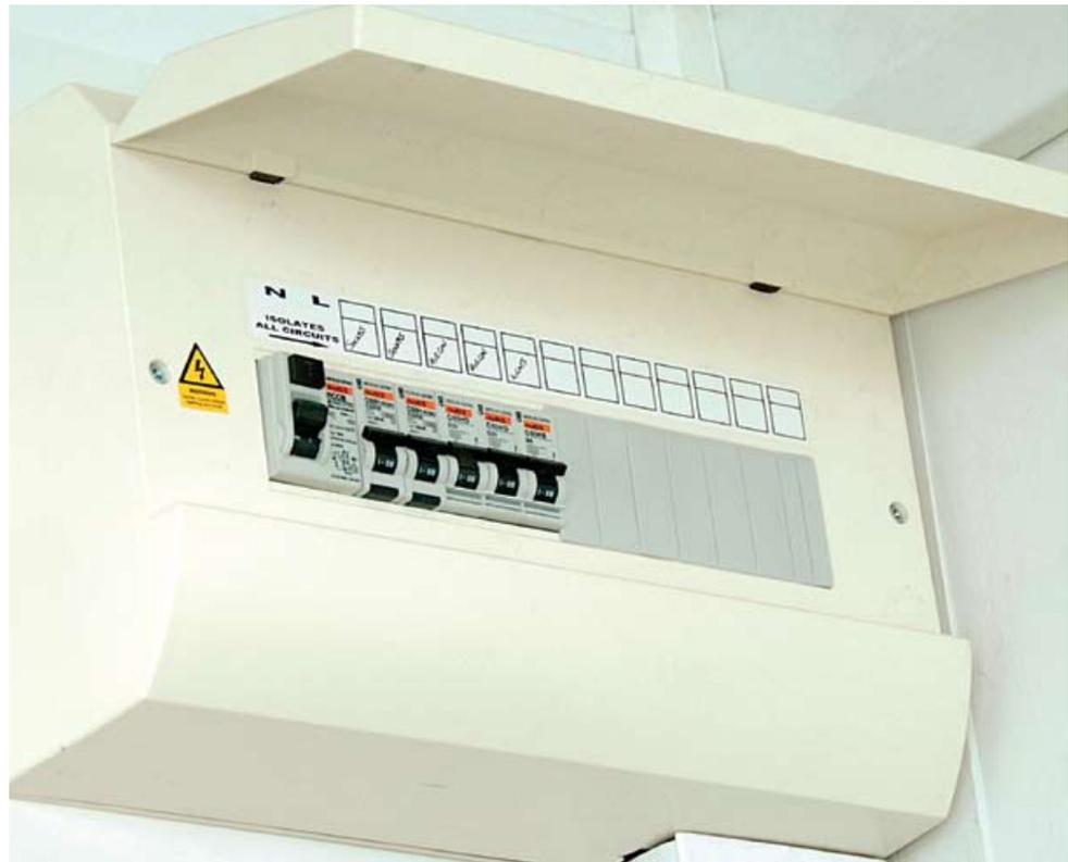
Figure 9 An RCD in a distribution board
