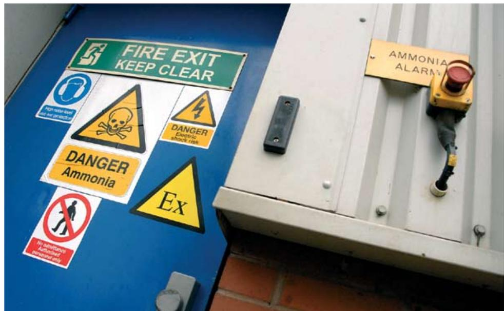
**Figure 56** An ammonia plant room emergency exit and alarm
