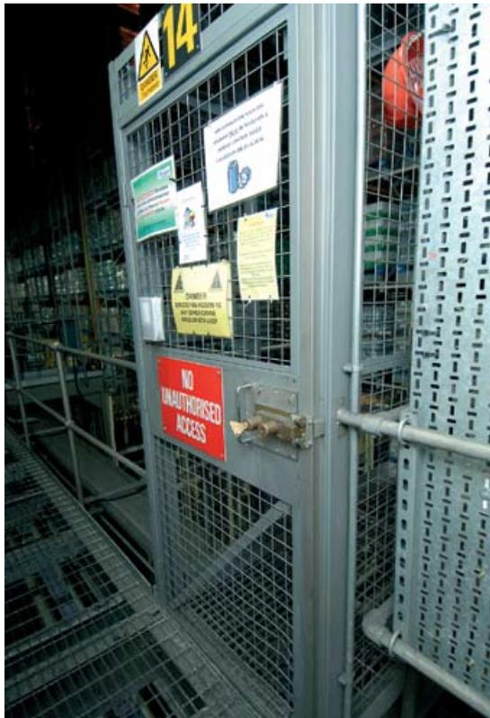
Figure 53 Interlocked access
